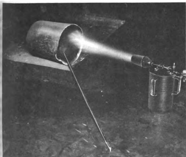
102.102 Figure 12-1. — Preheating the ladle.
